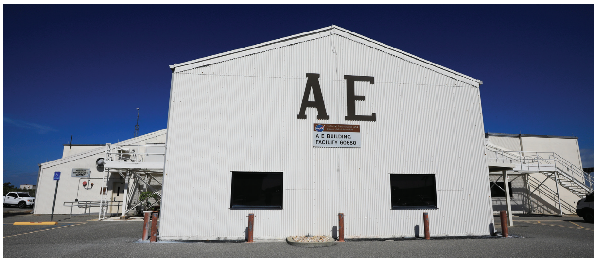
Hangar AE at Cape Canaveral Space Force Station in Florida houses control rooms providing real-time voice, data, and video information for expendable launch vehicle checkout and operations, and is used to support the uncrewed launch vehicle fleet. Photo credit: NASA/Ben Smegelsky
