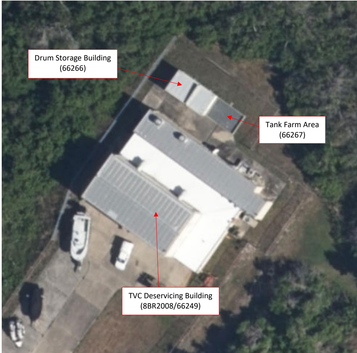
Figure 1. TVC Deservicing Building, Drum Storage Building, and Tank Farm Area.
