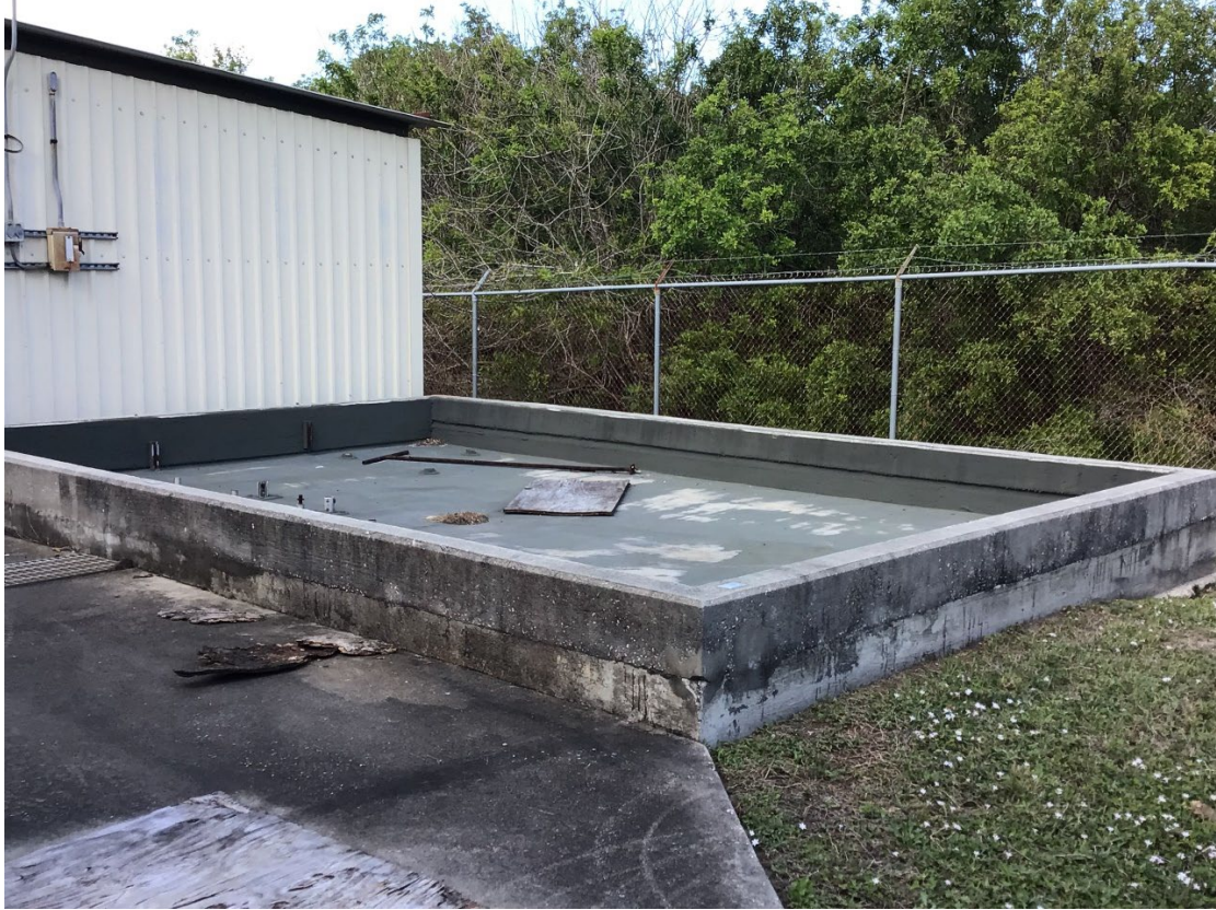
Figure 5. Tank Farm Area. Drum Storage Building is on the left.
