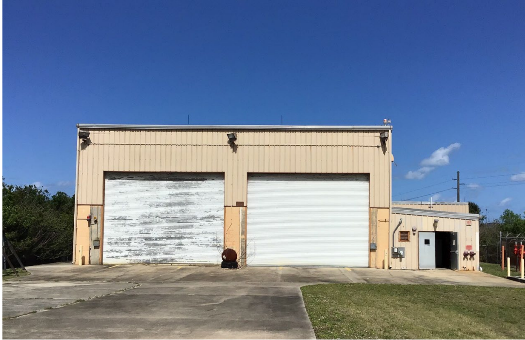
Figure 3. TVC Deservicing Building.
