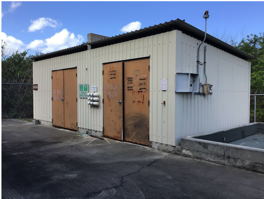
Figure 4. Drum Storage Building. Tank Farm Area is on the right.
