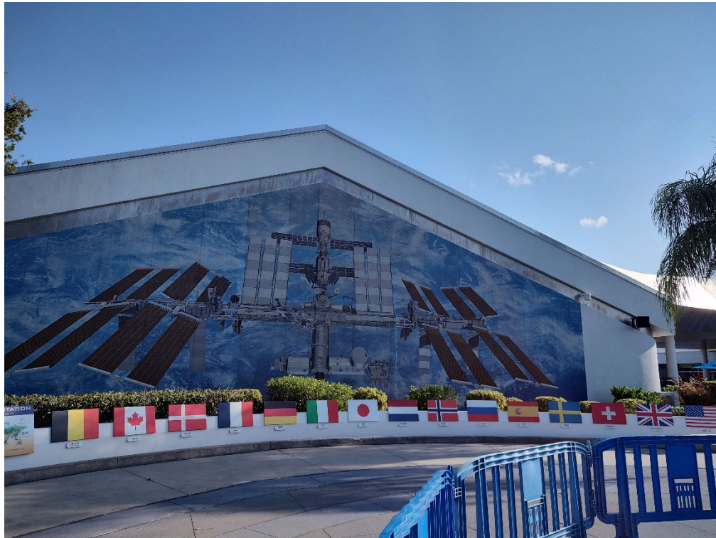
Figure 5. South Façade of M6-0409E Space Flight Exhibit
