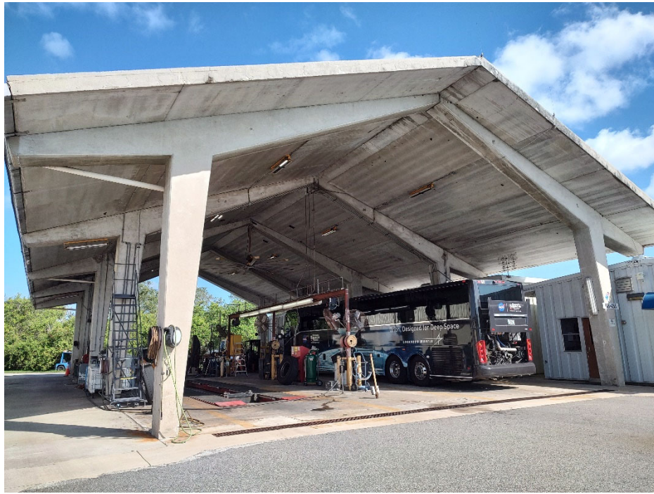
Figure 7. South Façade of M6-0455 Tour Bus Servicing
