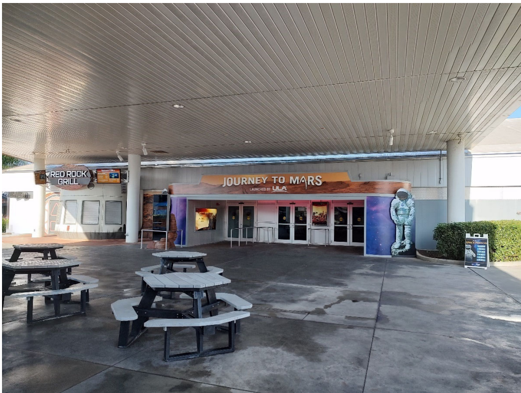
Figure 4. East Façade of M6-0409E Space Flight Exhibit
