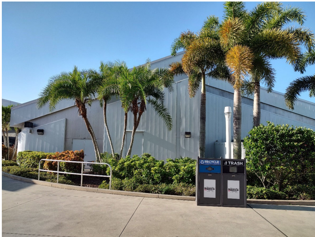
Figure 6. North Façade of M6-0409E Space Flight Exhibit
